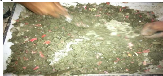
Fig-2: Mixing of E- Waste in Concrete
