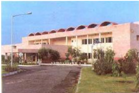
A view of the Administrative Block
