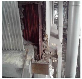
The total uninsulated area is 50sqm and the surface temperature is 400°C. The uninsulated areas cause surface heat loss. It requires insulation where
