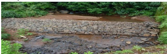
Fig No-10:- Mhasavandi Village Gabion Bandhara after development.
