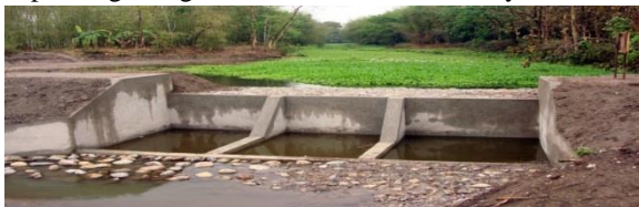
Fig No-09:- Mhasavandi Village -KT-Weirs after development.
