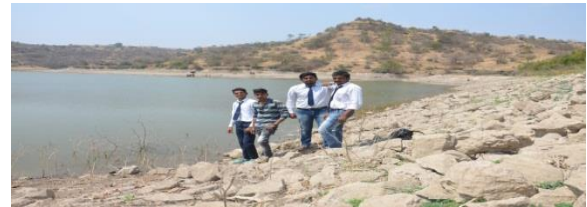
Fig No-11:- Mhasavandi Village Percolating Bandhara after development.
