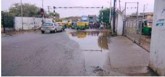
Figure 2. Water logging at kalol railway crossing.
