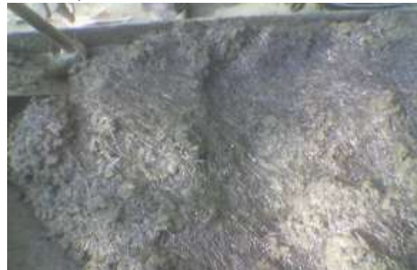
Fig 5 Mixing of concrete with steel fibres
