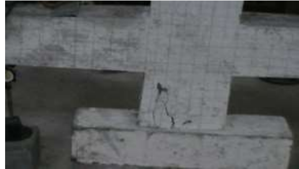
Fig 7 Failure of SFRC Beam-Column Joint
