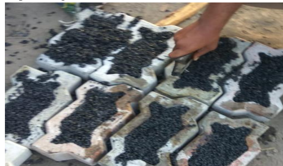
Fig. 3.3 Placing Mix bituminous on prepared Paver Block
