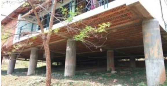
Fig 7: Cottages built on cylindrical concrete pipes
