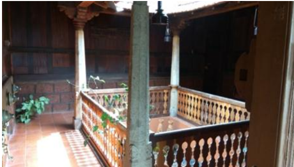
Fig 25: Open courtyard which allows natural light, air and rain water inside cottages
