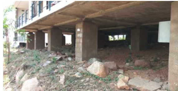
Fig 8: Cottages built on concrete blocks
