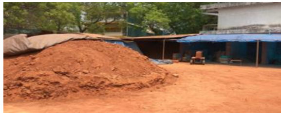
Fig 33: Soil for the production of CSEB being covered with plastic sheet
