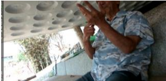
Fig 13: Bamboo baskets stuck to the underside of the RCC flooring.
