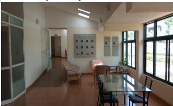
Fig 10: Natural day light obtained using large sliding windows and openings on roof
