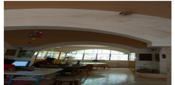
Fig 29: Inside view of the Office room
