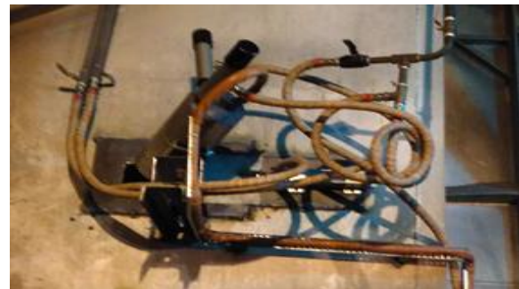
Fig. 12 : Onsite installation of the camera unit along with nitrogen cooling facilities.
