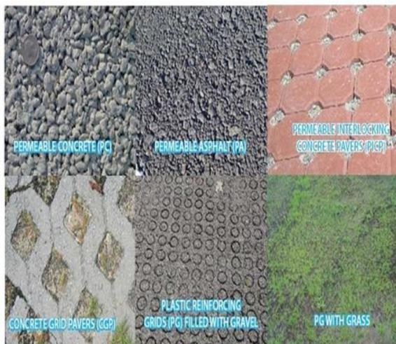
Fig – 1 Types of permeable pavement
