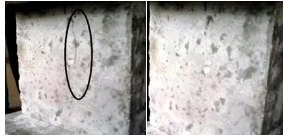
Figure 4: Crack healed concrete specimen with crack (left) & Healed Specimen (right)
