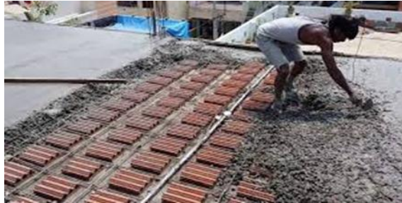
Fig[4]:- Filler Slab
