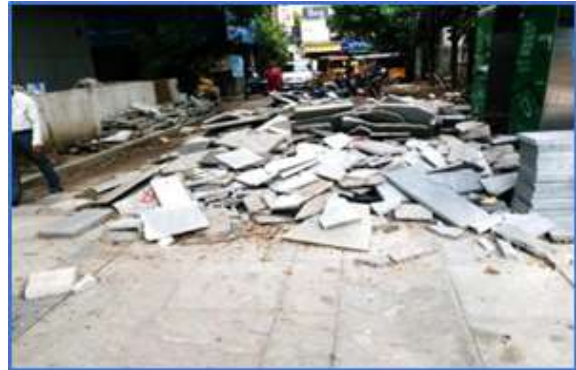
Collection of aggregates from demolished structure.
