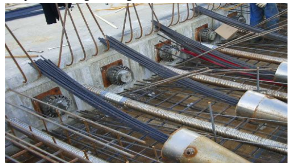
Figure 1: Bonded PT system
