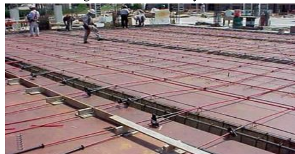
Figure 2: Un-bonded PT system
