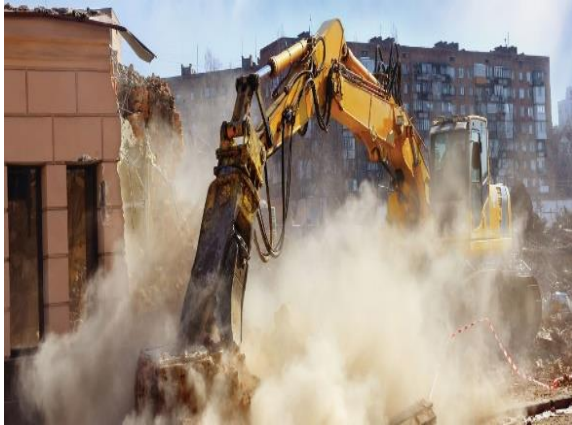
Figure.1: Dust at demolition site
