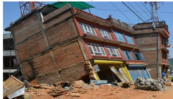
Fig 1.1 Example of foundation failure during 2015 Gorkha earthquake in Nepal
