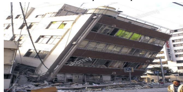
Fig: Example of foundation failure during 1995 Kobe earthquake in Japan
