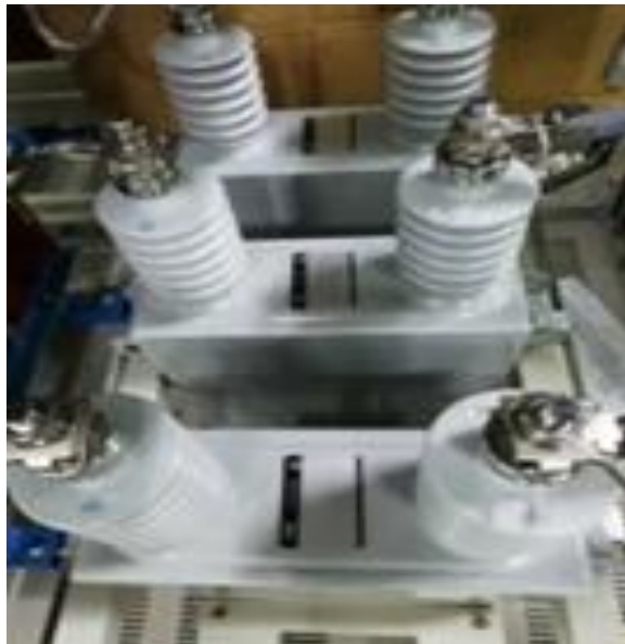
(e) CAPACITOR BANK
