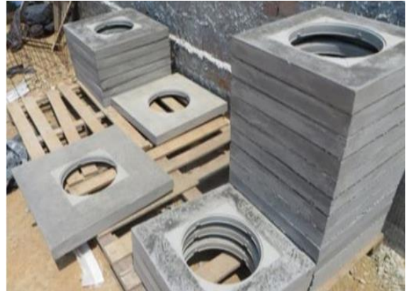
FIGURE 03: Covers for inspection boxes molded in situ.
