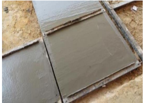
FIGURE 04: Covers for inspection boxes molded in situ.
