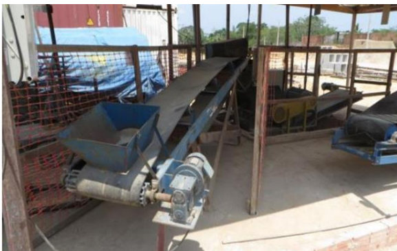
Figure 12: Waste Shredder for Aggregate Transformation.
