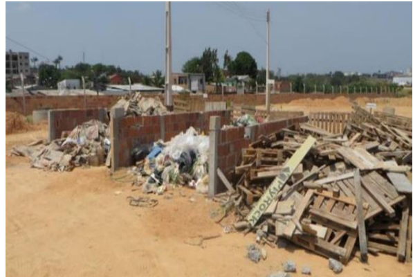
FIGURE 09: Waste conditioning bays.
