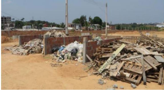
FIGURE 13: Management of Residues of Company correctly practicing the disposal of waste.
