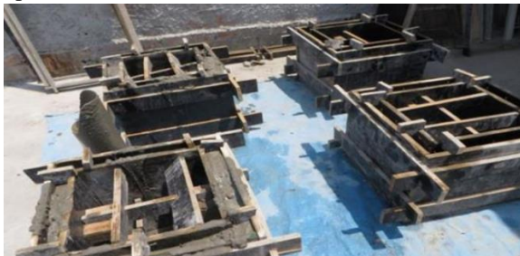
FIGURE 01: Preparation of forms for molding inspection boxes.
