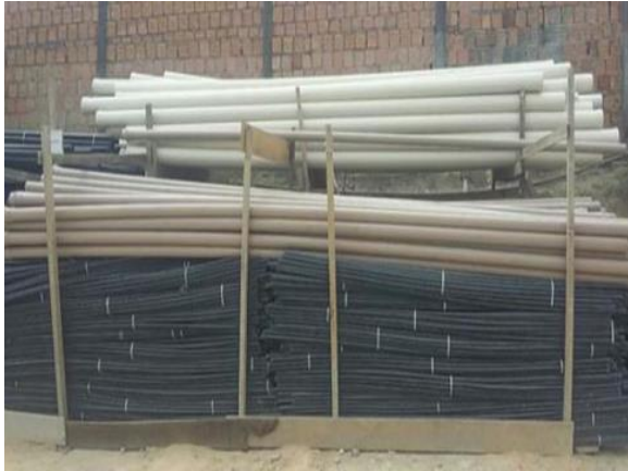
FIGURE 05: Proper storage of tubes and steel bars.
