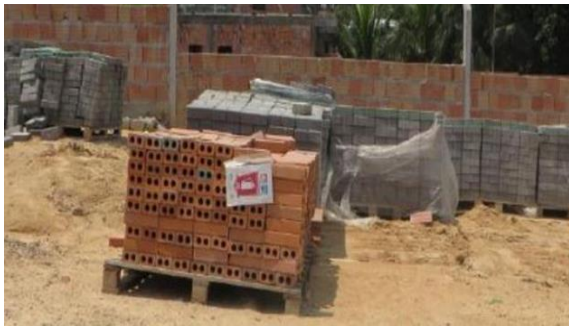
FIGURE 06: Proper storage of building blocks.
