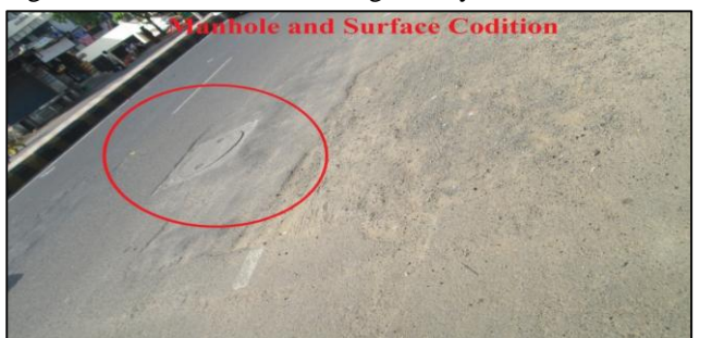
Figure 5: Manhole and surface condition
