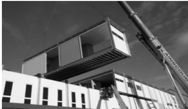
Figure II: Modules being lifted with crane
