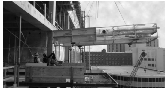
Figure IV: MEP Multi-trade racks site installation, Source: Modular services company
