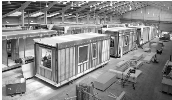
Figure I: Modules being prefabricated in factory
