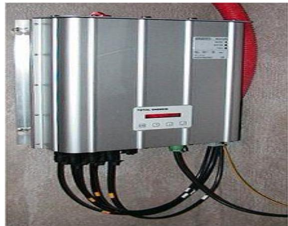
*Inverter for grid connected PV
