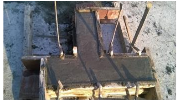
Fig.3 Casted Specimen of RC Beam-Column Junction with Grade of M30
