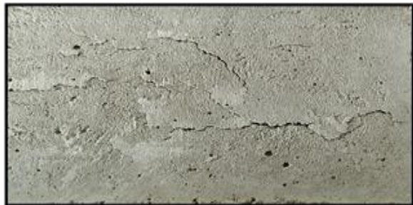
Fig. 7 – Crack Observation
