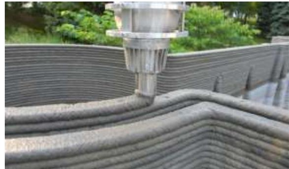
The above image shows the printing of wall through 3D printer and its easy to make at less cost. 3D printing can save a lot in infrastructure, it saves approx 30% to 60% waste and decrease production time by 50 – 70 percent and also it affects labour cost in between 50 – 80 percent of savings.[5]
