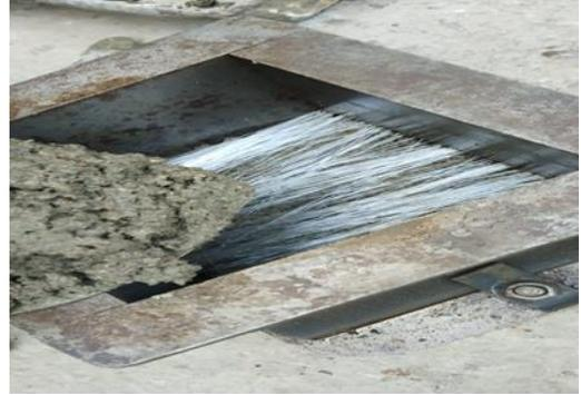
Fig No.6.Placing of Plastic optical fibres
