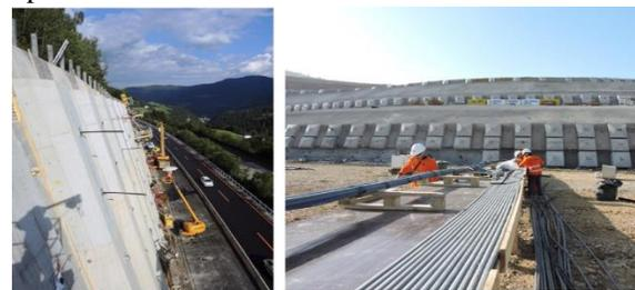
Figure 7. Slope stabilization using ground anchors for retaining walls at highway (left) and at a refinery (right)
