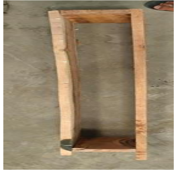
Figure 3. Formwork of Beam
