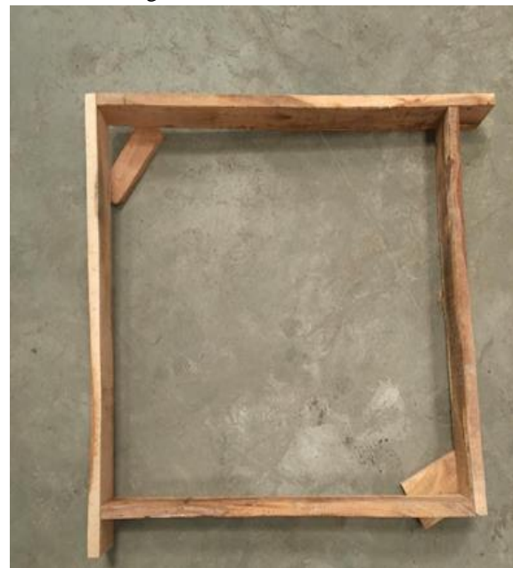
Figure 4. Formwork of slab
