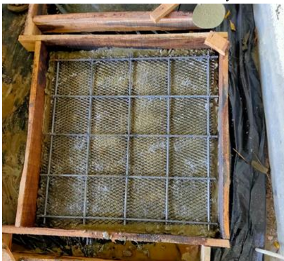
Figure 7. Steel reinforcement in Slab bonded with geosynthetics.
