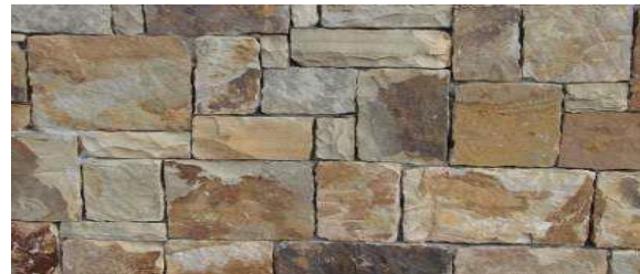
Fig. No.3 – Ashlar Stone masonry
