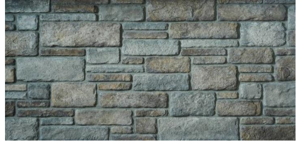
Fig. No.2 – Stone masonry
