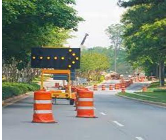
Fig. 2 Roadside Hazards for safety
