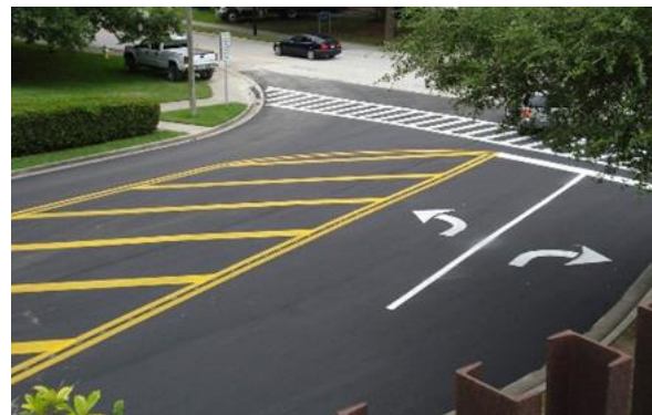
Fig. 1 Markings done for safety
