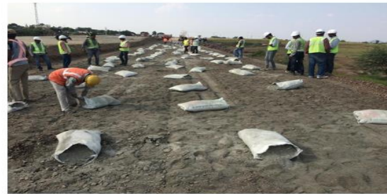
Figure 5: Process of Site blending- Manual mixing of Additives at directly at site
