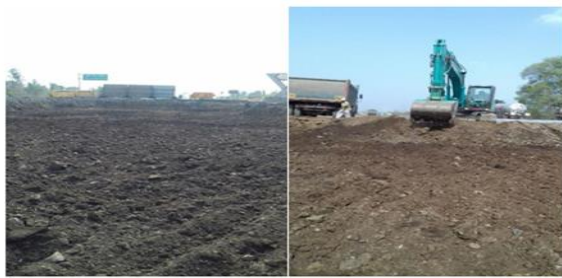
Figure 2: Removal of BC Soil at Vita Kokrud Section of SH 150
