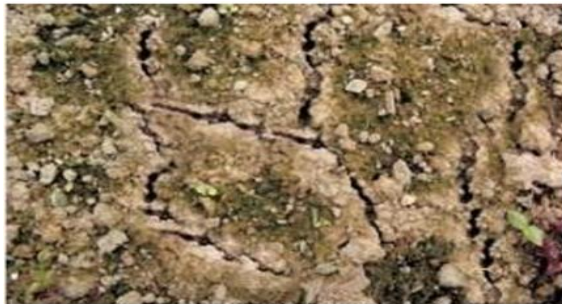
Figure 1: Crack in BC Soil
