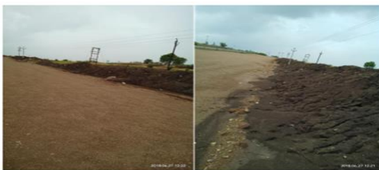
Figure 2: Removal of BC Soil at Vita Kokrud Section of SH 150
