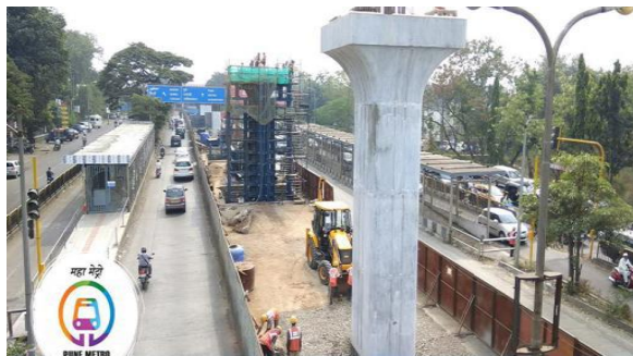
Fig. Pier at Nagpur Metro Construction Site
