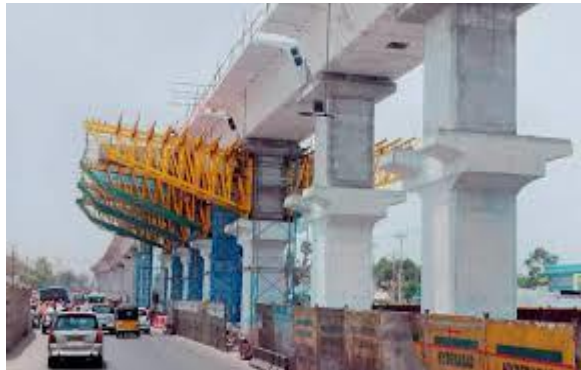
Fig. I girder platform level
