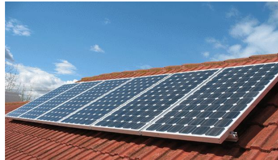
Fig. Solar Panel
