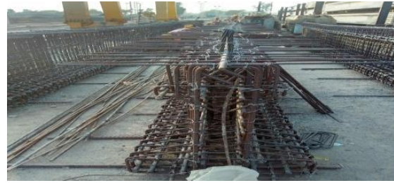
Fig. Reinforcement of I girder
