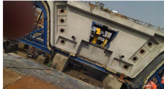
Fig. Segment of Box Girder
