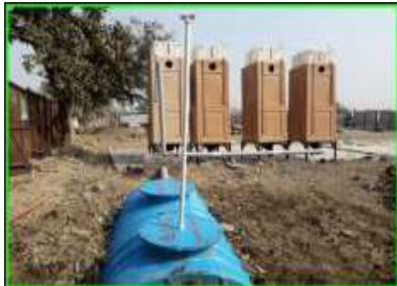
Fig .Bio Digester at Depot
