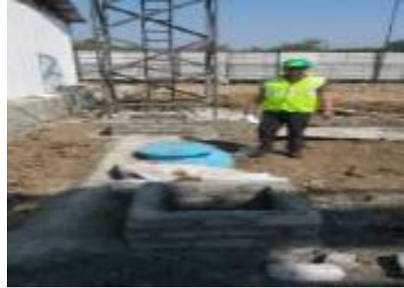
Fig. Bio Digester Installation at Office Camp
