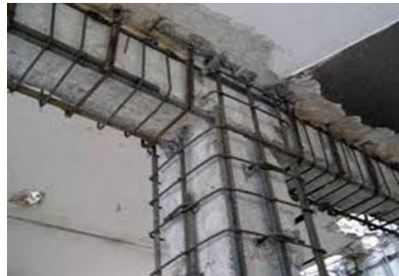
Fig. 1- Beam jacketing
