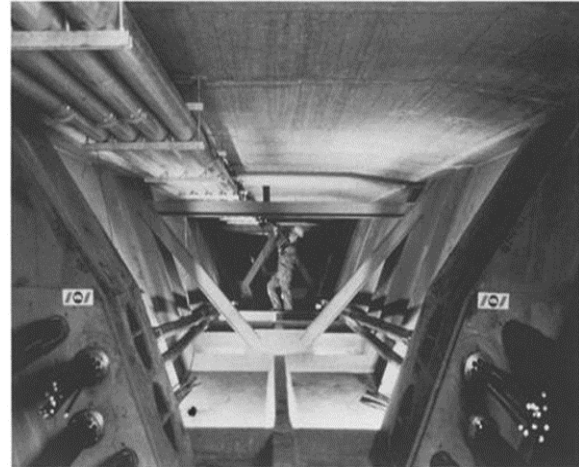
Figure 1.8 Prestressed double-tee roof beams.
