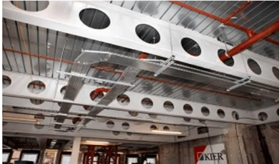
FIG-1.1 CFS SECTION WITH PERFORATION
