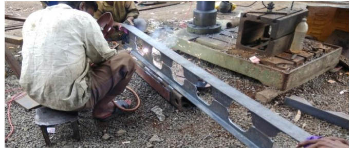
Figure No. 3 Welding of castellated beam III) Grinding -
