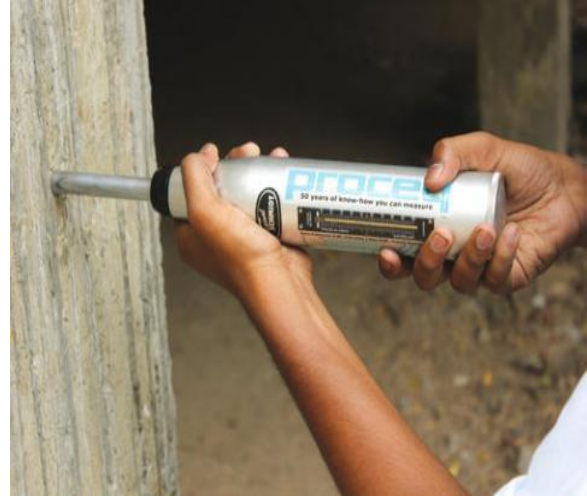
Rebound hammer test
