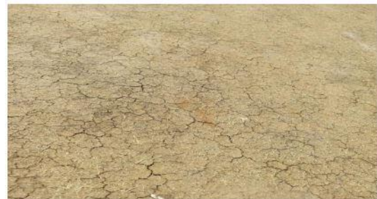
Figure 3: Cracks due to excess water in pitch
