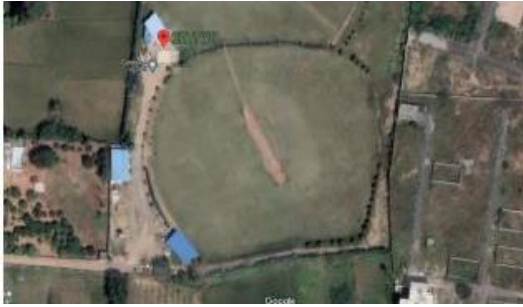
Figure 5: Aerial view of ABRR cricket ground located at Balapur, Hyderabad
