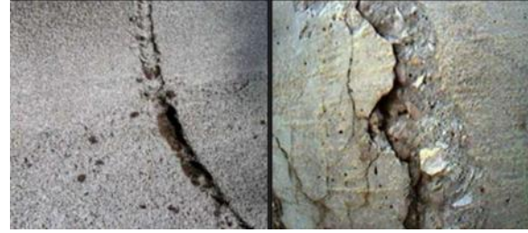
Fig (5):Welding Defect Fig (6):Material Loss
