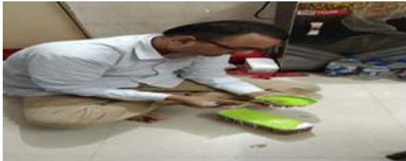
Figure 2 Application of Chalkboard Paint on Lime Plaster
