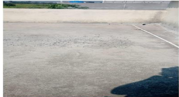
3) Top View of Terrace Level Without Water Proofing, No leaks Problem
