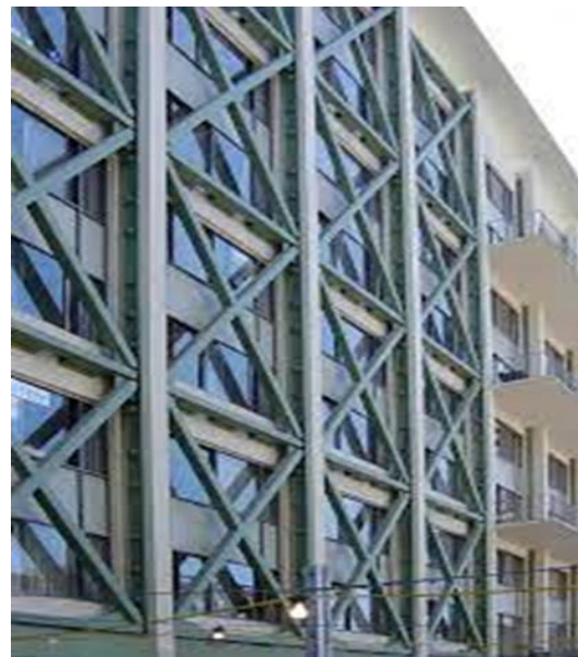
fig.1. Use of friction dampers in building
