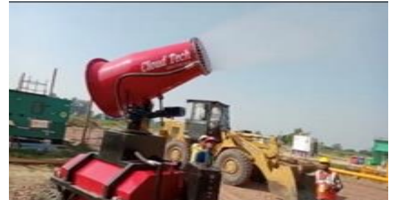
Photo 6, dust mitigation by Anti-smog gun
