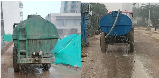
Photo 5, water sprinkling by the tanker
