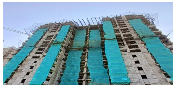
Photo 7, Green net fixing on building face to prevent movement of dust
