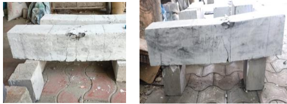
FIG 5 Crack Pattern on Beam
