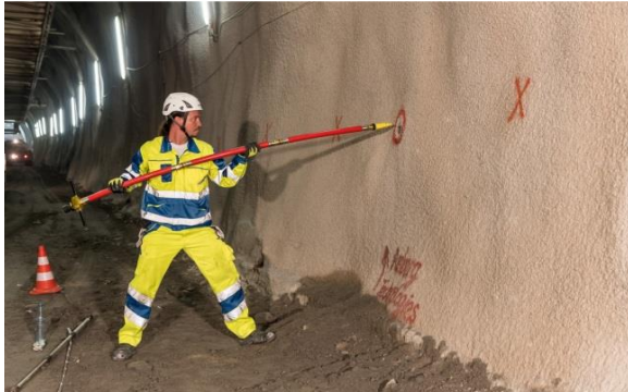
Figure 3 (i). Installation of receivers and recording unit to TSP campaign.
