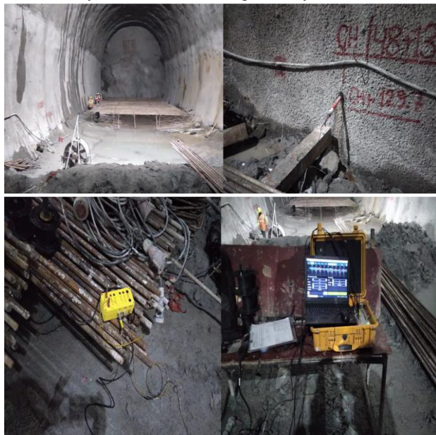
Figure 6: Progressive photographs during TSP operation.
