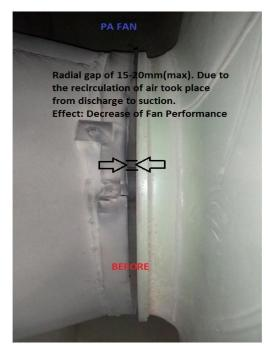
The radial gap between inlet cone and impeller eye is 20mm causes recirculation of air. the gap should be reduce or seal with copper sheet.
