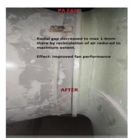
Copper sheet is a soft, malleable and ductile metal. It suited for sealing the gap because if the copper sheet damage it breaks into small pieces it does not causes any damage to the fan
