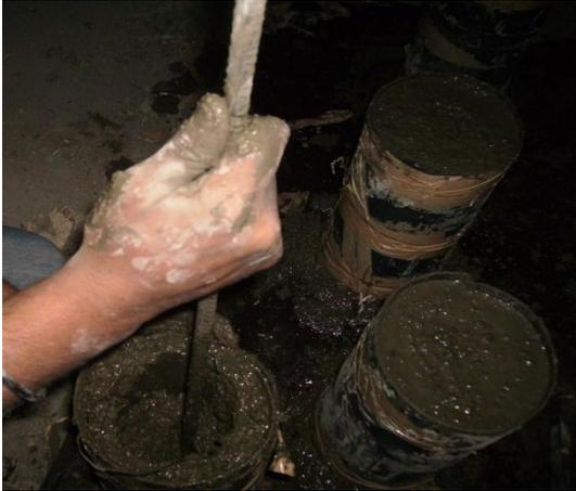
Placing of M10 concrete in core and Mortar at periphery
