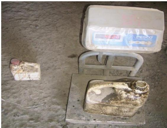
Weight batching of water and Admixture
