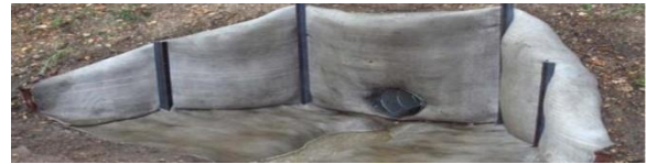
Fig. 3: - Culvert Protection
