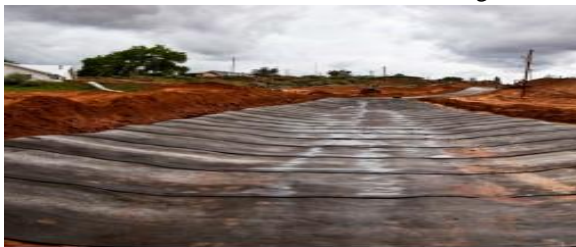
Fig. 8: - Tank Lining
