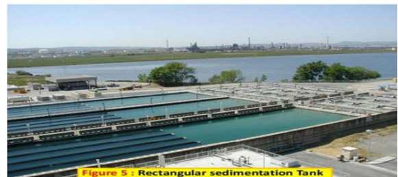
Figure 5 : Rectangular sedimentation Tank
