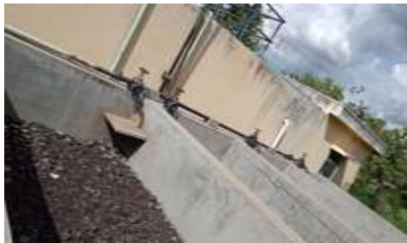
Sludge drying beds
