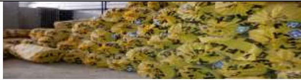
Fig. 6.A.3.11 Thermal Insulation Materials must be covered
