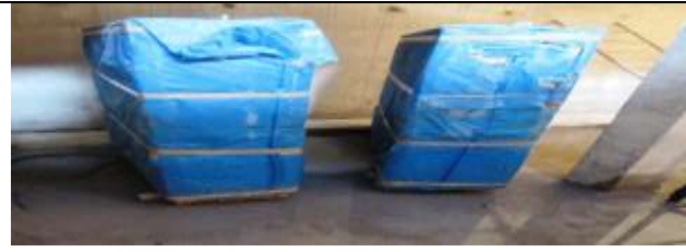
Fig. 6.A.3.11 Thermal Insulation Materials must be covered
